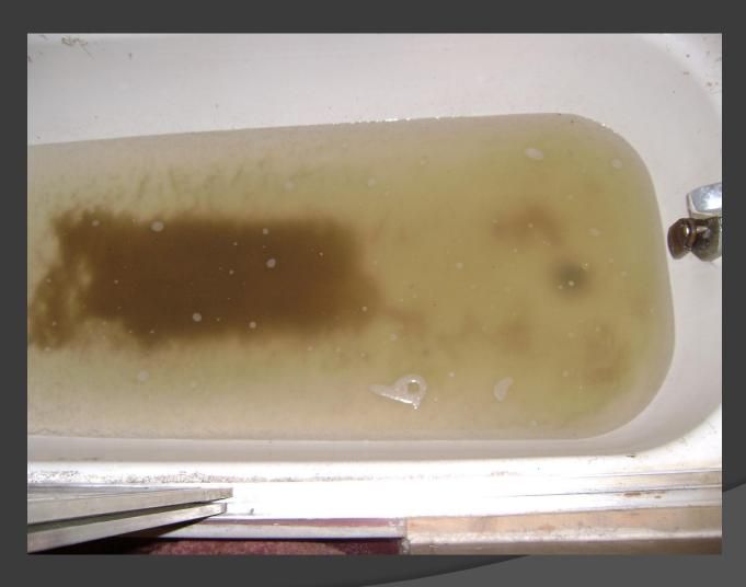
Damage caused in a resident's home by a sewer blockage. This backup was due to wipes/rags and grease in the City sewer main.
