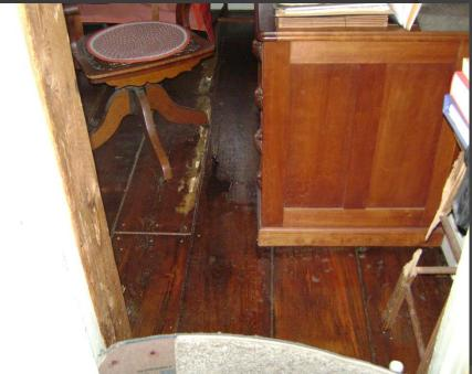
Sanitary Sewer Overflow (SSO). SSO's occur when sewer mains are clogged preventing flow through the pipe. Water will find a path of least resistance either in a home or outside environment.
