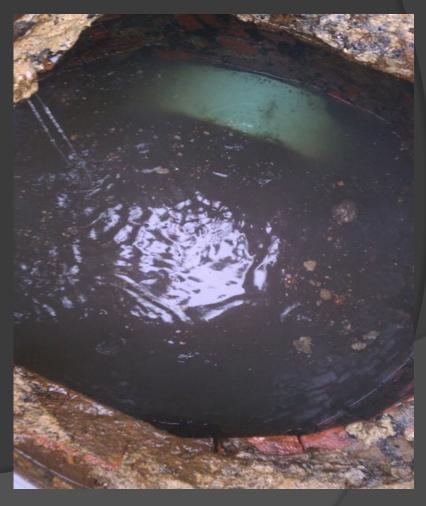
Scotland Rd lift station, grease enters the wet well picture left, it forms and hardens around the equipment, pumps, transducers, etc. picture right, also rags/wipes combined with grease will cause failure at the stations. This station pumps 60,000-80,000 GPD.
