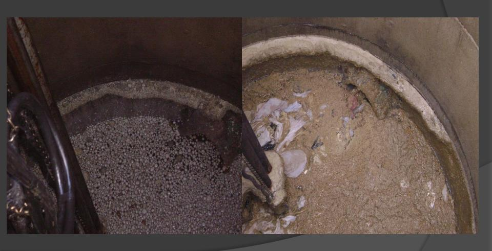
SEWER BACK UP! This photo was taken at a resident's home. The bath tub in the home was filled with sewage due to City sewer main blocked with grease and rags/wipes.
